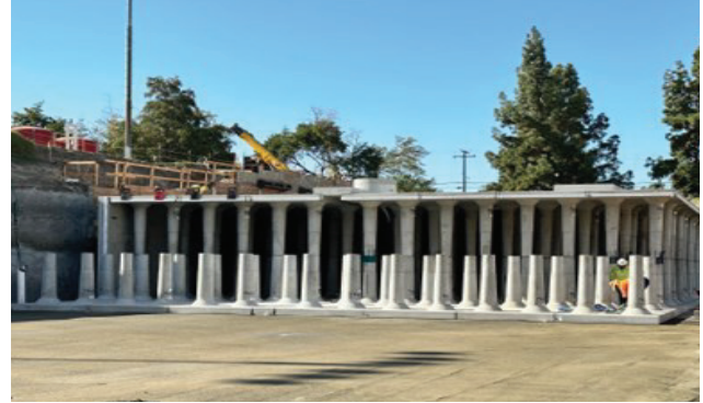
StormPrism System 6' to 14' (Interior) Double Stack—Integral Bottom Slab
