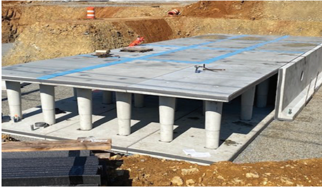
StormPrism Module 4' to 7' (interior) Single Stack—Top Section on Concrete Base Slab
