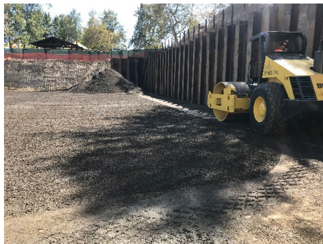
Fig. 1 – Roller compacting the subgrade of a detention system
