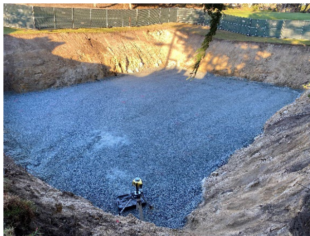
Fig. 3 – Completed subbase of an infiltration system
