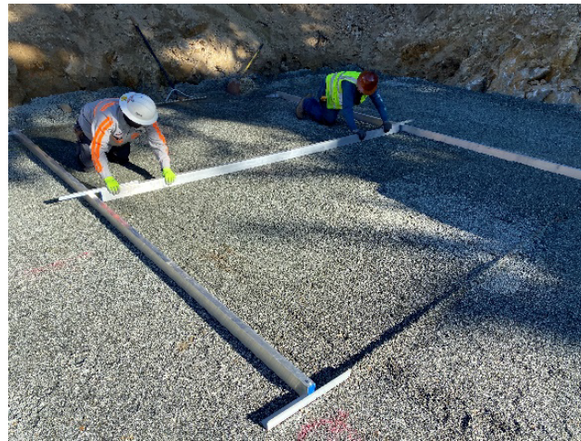
Fig. 4 – Hand screeding the base of a small infiltration system
