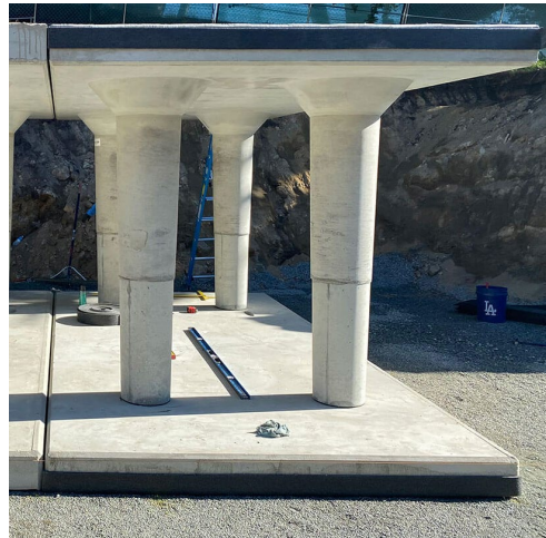
Fig. 11 – Fastflex spacer glued to top deck and Nomaflex glued to floor of a single level system
