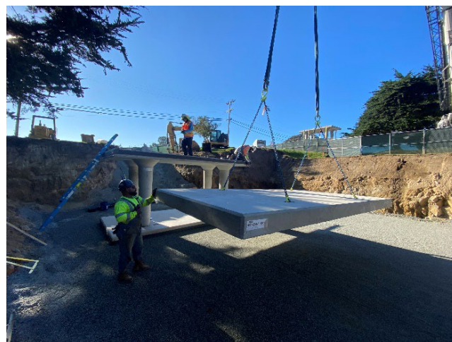
Fig. 5 – Recommended rigging
