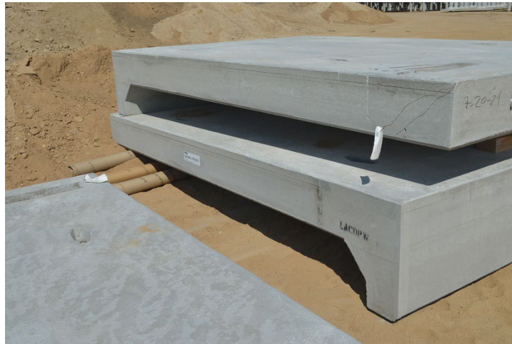
Fig. 6 – Wall components stored on-site in horizontal orientation
