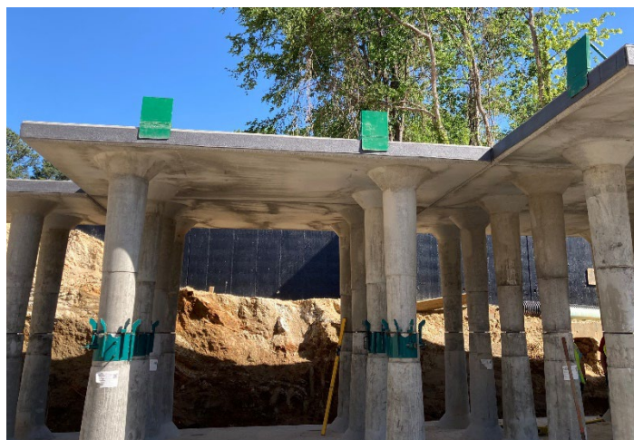
Fig. 12 – Double level system with metal guides at legs and shoehorns at top deck
