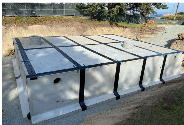
Fig. 13 – System sealed with polymer wrap and L-brackets
